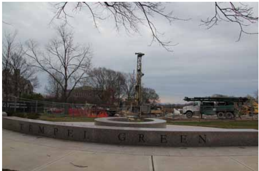
Geothermal drilling on Tempel Green
